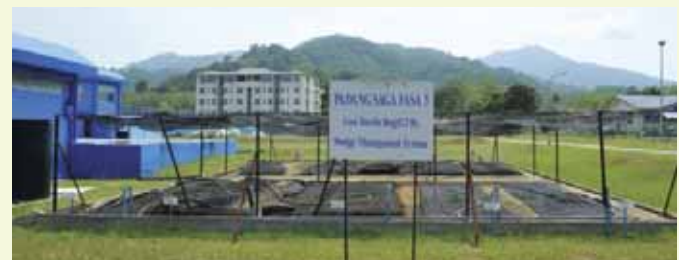
Sludge Dewatering Bag
